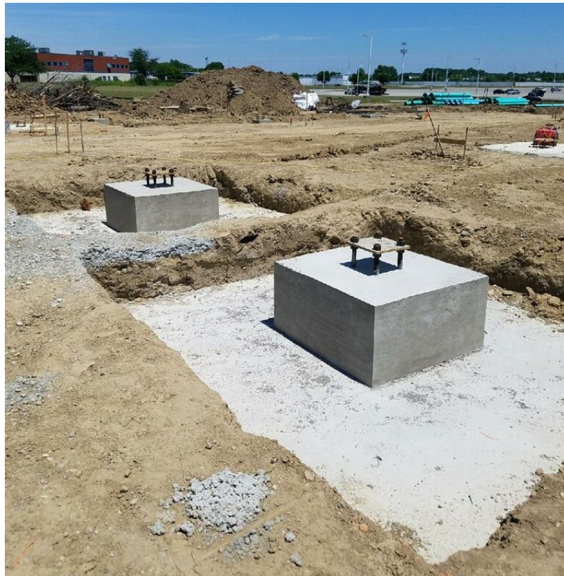
Project Site on June 6, 2018 View of the large footing pad with concrete pier and steel column anchor bolts.
