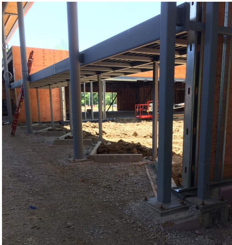
Project Site on June 5, 2018 View of the saw-tooth seating area off the Main Concourse.
