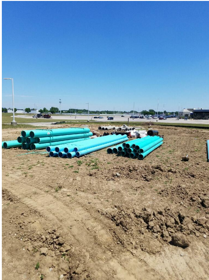
Project Site on June 6, 2018
